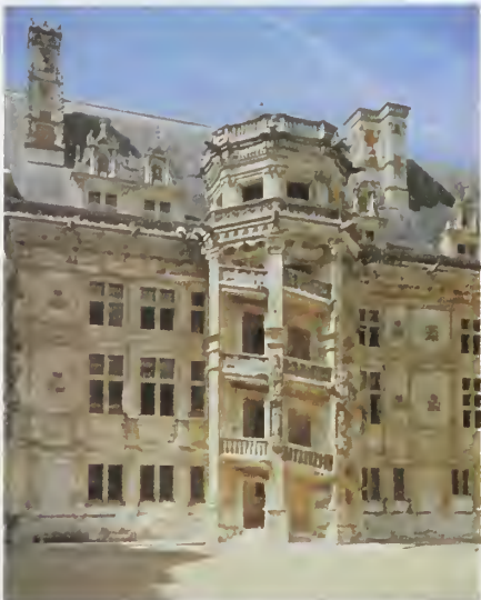
The château at Blois, Fr., with the Francis I exterior staircase Club Ins
